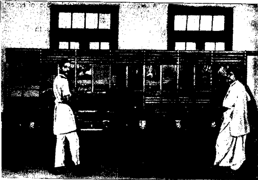
ERRECTION OF C. B. SWITCH BOARD BY THE MECHANIC OF THE DEPARTMENT AT THE TIME OF CHANGE OVER FROM MAGNETO TO CENTRAL BATTERY SYSTEM.
